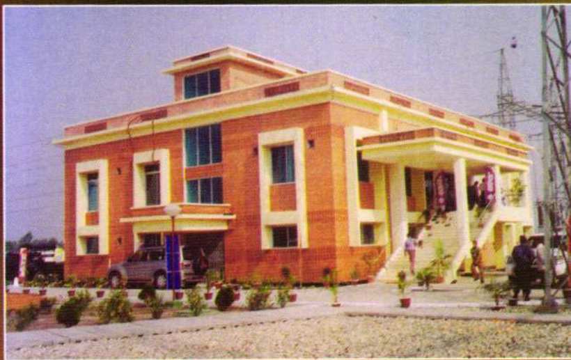
Control Room Building of Sirajganj 230/132 kV Substation.
