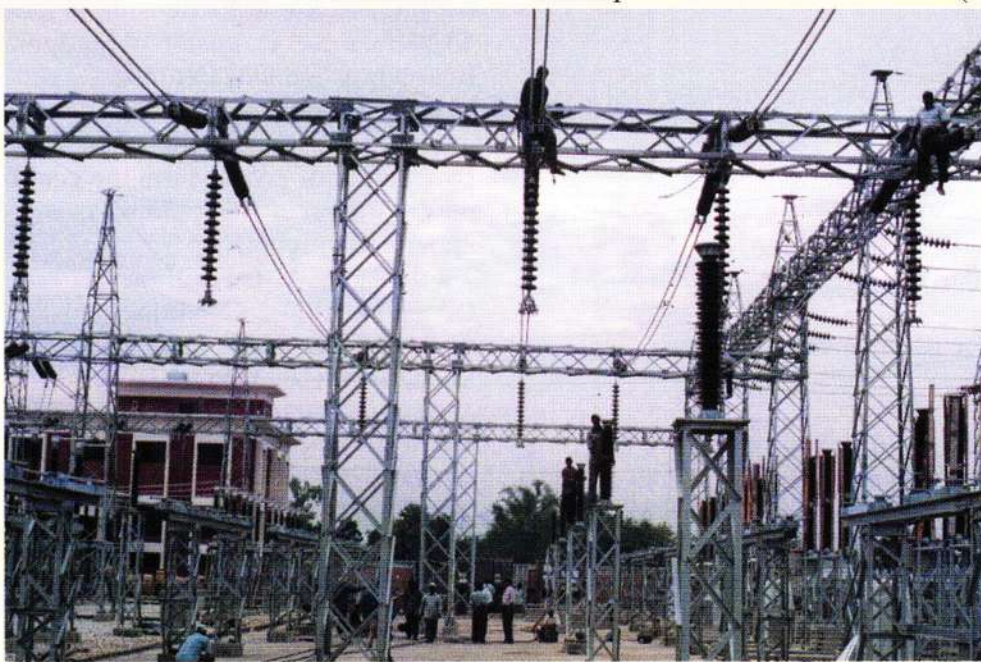
Partial view of Barapukuria 230/132 kV Sub-station under construction
