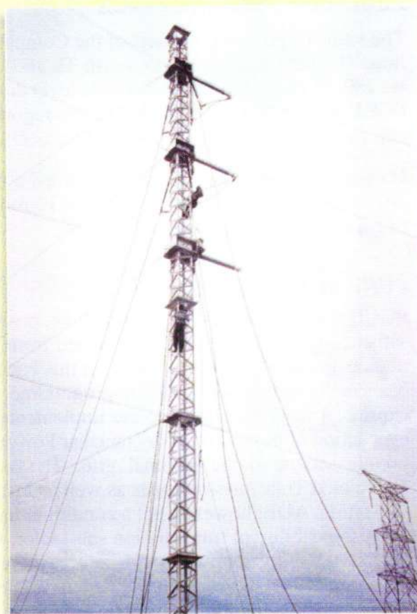
Emergency Restoration System (ERS) erected at Aminbazar Sub-station site.
