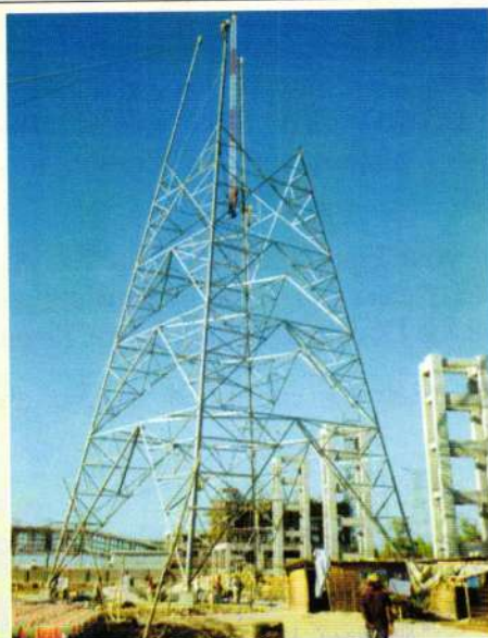
Erection of Terminal Tower in progress at Barapukuria Sub-station.
