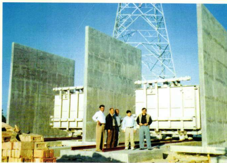
Installation of transformers at Barapukuria Sub-station.
