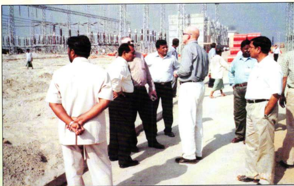
Partial view of Aminbazar Sub-station under construction.
