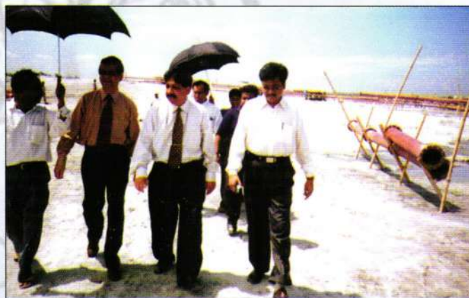
Site development for Aminbazar 230/132kV Substation
