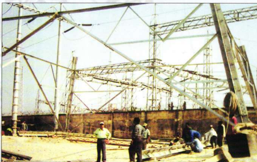
Tower erection for Hasnabad-Aminbazar-Tongi 230kV Transmission Line
