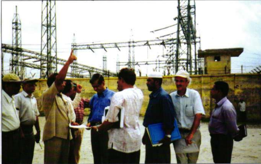
Inspection of 230kV Terminal Tower erection site near Hasnabad 230/132kV Substation
