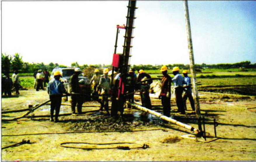
Foundation work in progress for erection of Tower for 230kV Hasnabad-Aminbazar-Tongi Transmission Line
