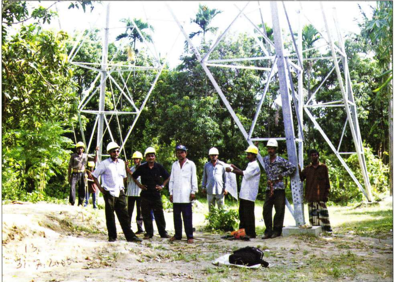
230 kV Tower erection in progress for Meghnaghat Power Station Associated Transmission Lines Project
