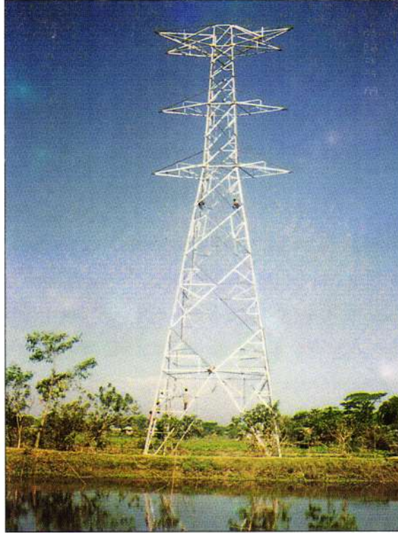
Erection of 230 kV Tower for Meghnaghat Power Station Associated Transmission Lines Project
