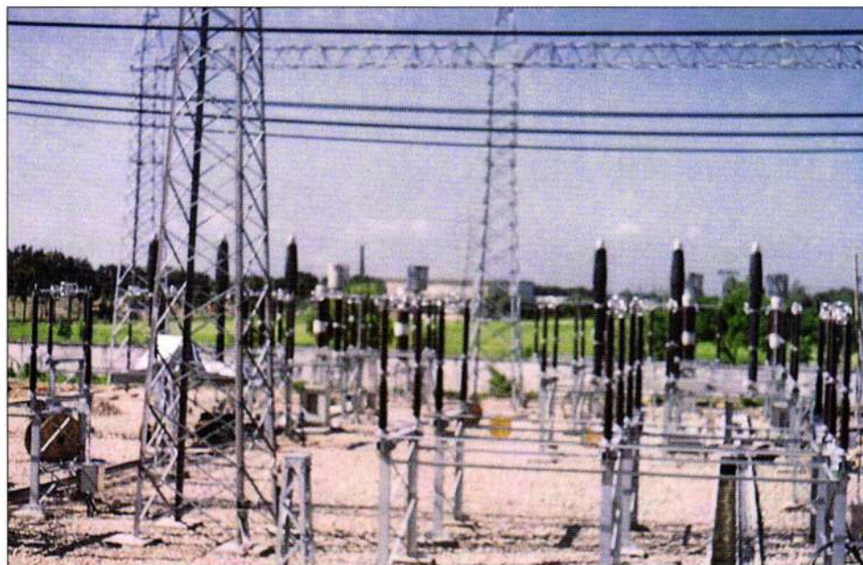
Extension work in progress at Comilla (North) 230 kV Substation
