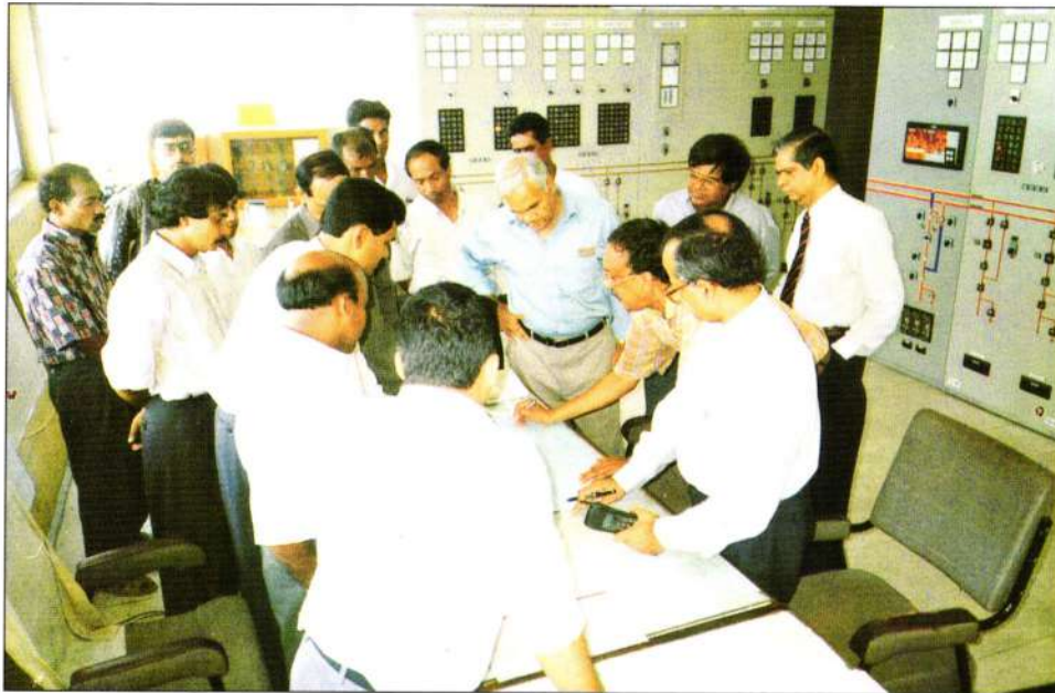
Chairman visiting Comilla (North) Substation
