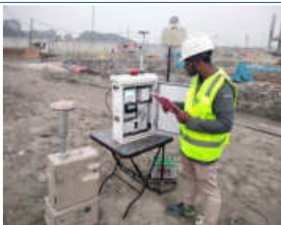
AQ39 Near 132/33 kV GIS substation at Maheshpur
