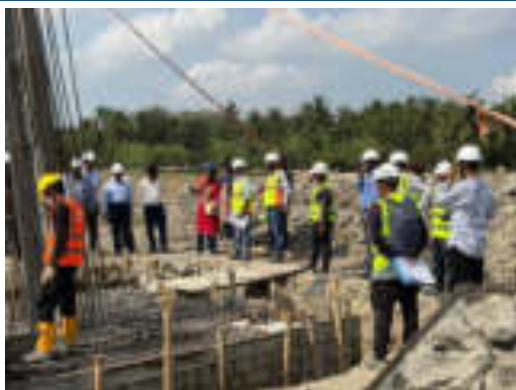
Erection observation of river crossing tower in SRTL
