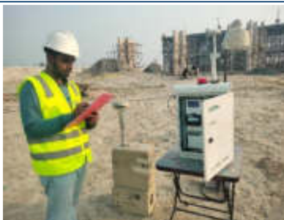
AQ41 Near 132/33 kV GIS substation at Manirampur
