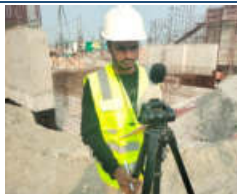
NL42 Near 230/132/33 kV GIS substation at Rupsha
