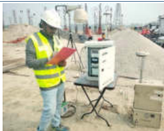
AQ40 Near 132/33 kV GIS substation at Meherpur
