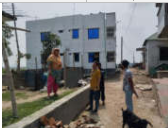
Package 5- Kaliganj Substation
