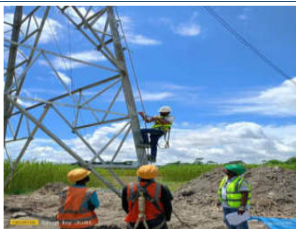
Erected Tower of Gopalganj-Shibchar 230 kV Transmission Line
