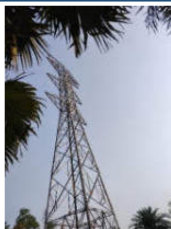
Erected Tower of Kaliganj- Maheshpur Transmission Line
