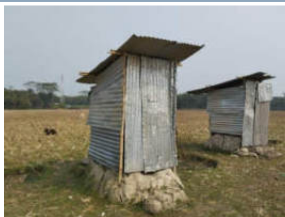
Temporary Toilet facilities at site
