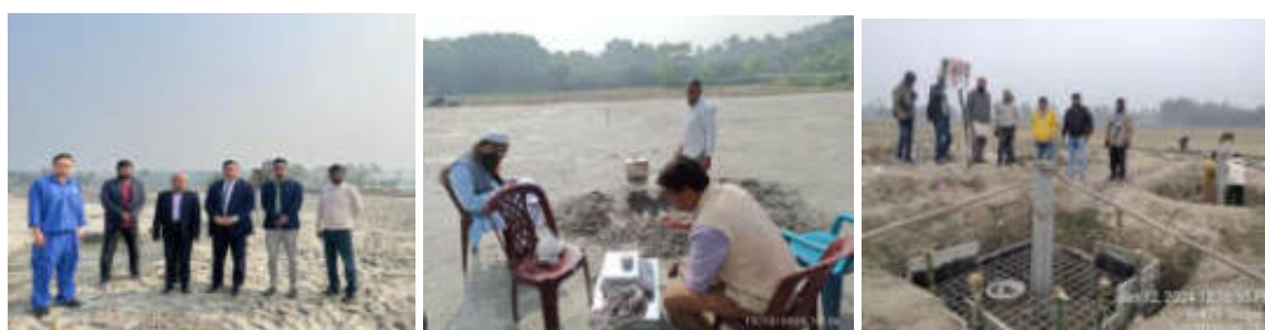
Inspection of land development, compaction test and Transmission line construction activities
