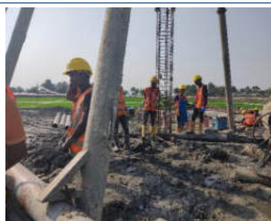
Piling Work at Satkhira-Rupsha 230 kV Transmission Line
