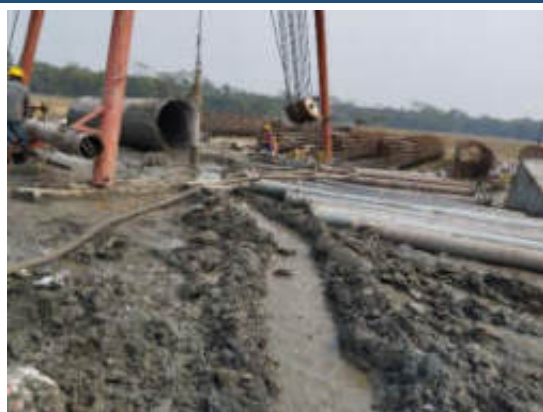
Piling Mud Drain
