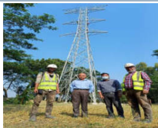
Erected Tower of Gopalganj-Shibchar 230 kV Transmission Line
