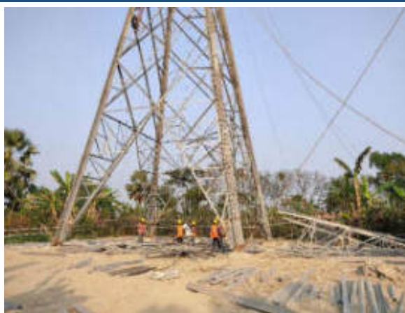
Erected Tower of Satkhira- Rupsha Transmission Line
