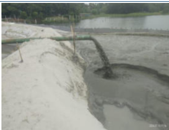
South Side of Purbachal Substation
