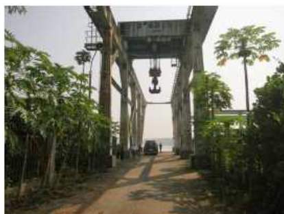
Whole-view of the cargo-handling facility (route width is 5400mm).
