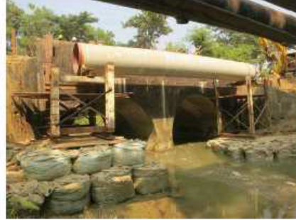
Bridge conditions: Concrete arch.
