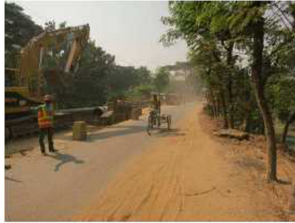
JICA work on water supply piping was being done at the time of the survey.
