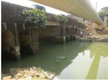
Bridge conditions: The piers are made of bricks.
