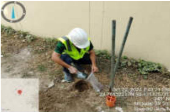
SQ-3- Non-agricultural land, Near the Substation Area of Aftabnagar
