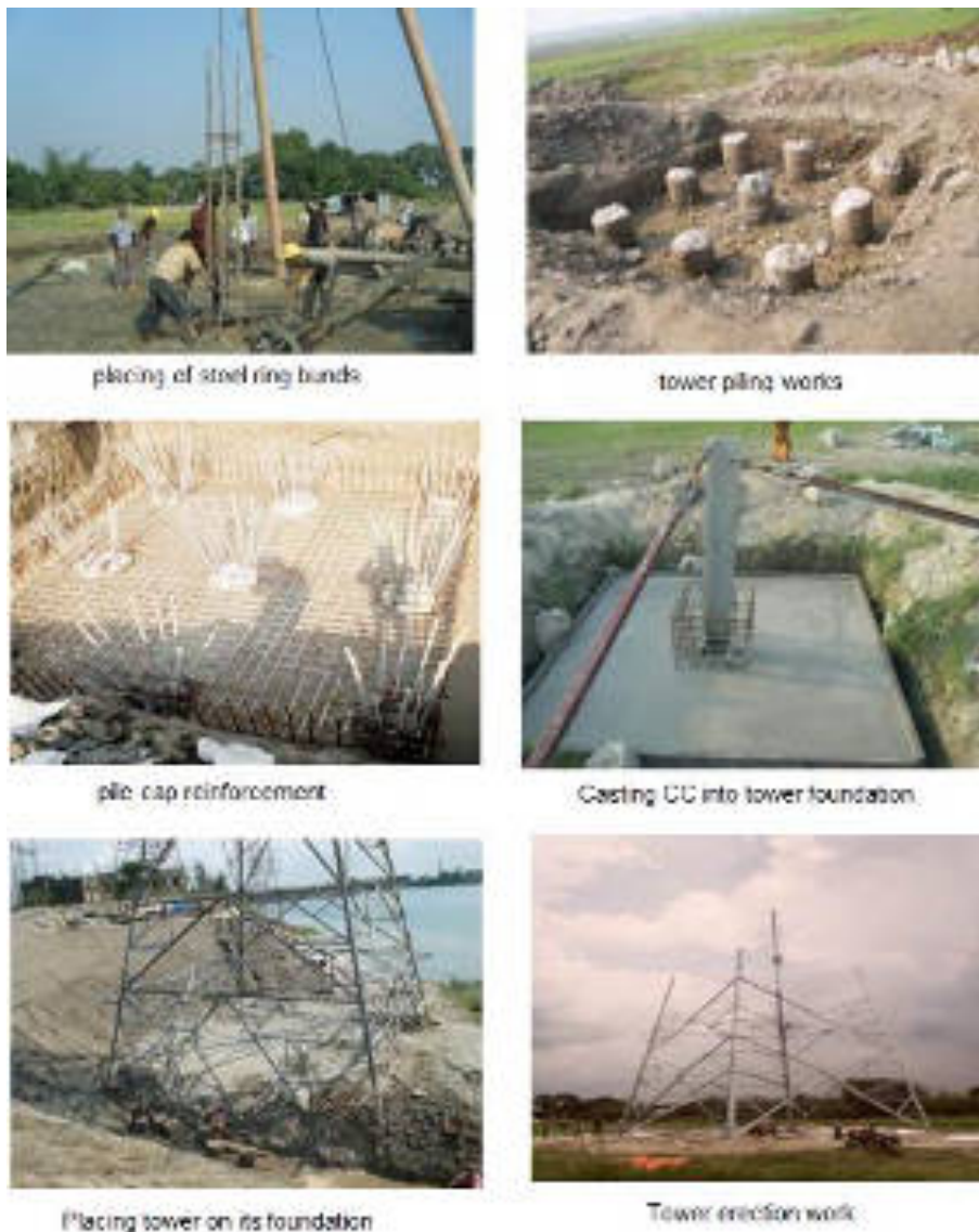
Figure 3-5: Associated Civil Works for Transmission Line Installation
