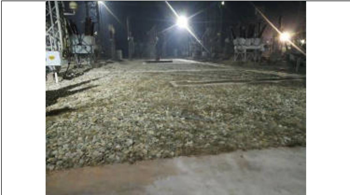
Plate 3.19 The land allocated for the bay extension
