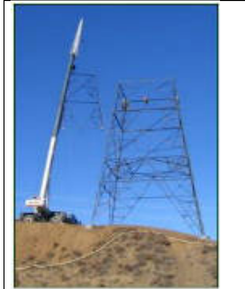
A crane carrying the top section of an LST for installation
