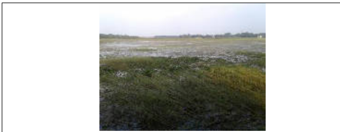
Plate 3.1 Land identified for the construction of Kaliganj (Gazipur) substation
