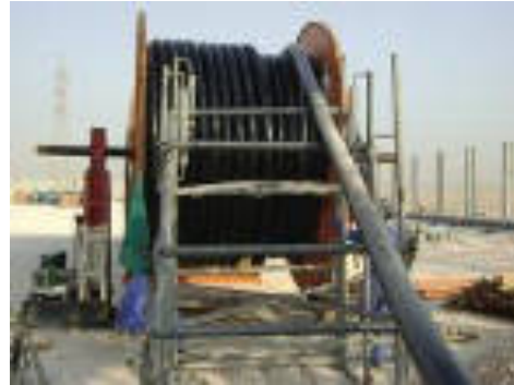
Figure 3-3: Placement of cable drum and correct method of pulling
