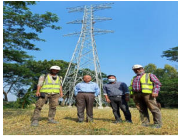
Erected Tower of Gopalganj-Sibchar 230 kV Transmission Line
