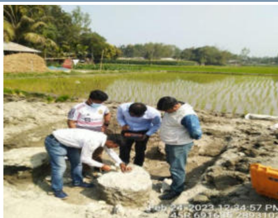
Pile Integrity Test at Domar-Hatibandha 132kV Transmission Line
