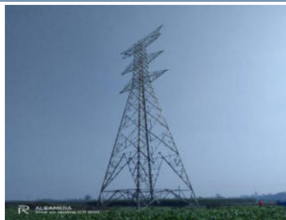
Erected Tower of Purba Sadipur-Domar 230 kV Transmission Line
