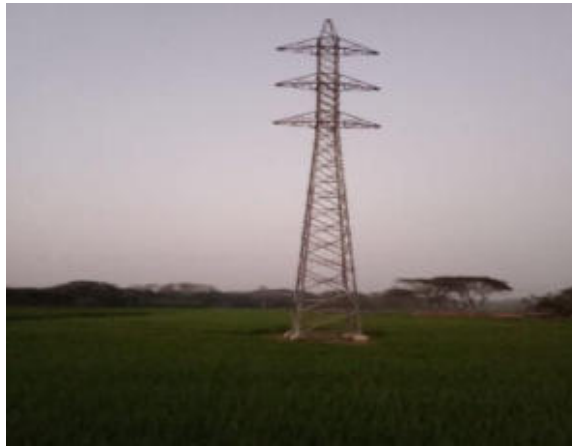
Erected Tower of Satkhira-Manirampur 132 kV Transmission Line
