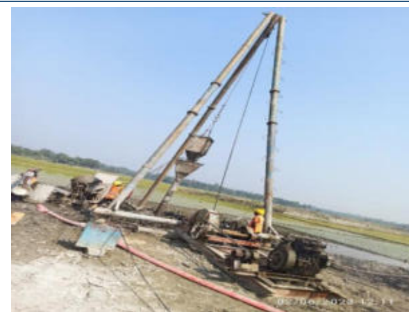
Piling Work at Satkhira-Rupsha 230 kV Transmission Line
