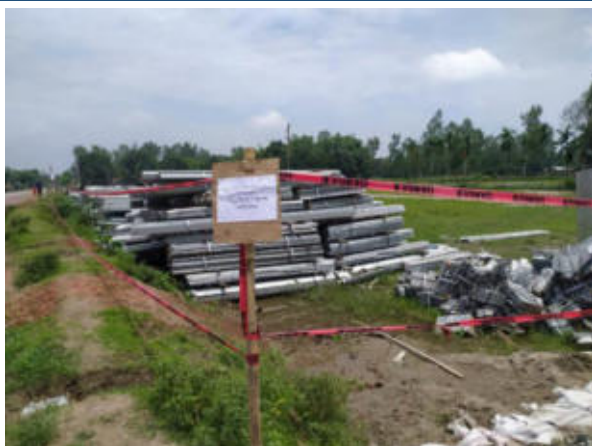
Materials stored at the designated area
